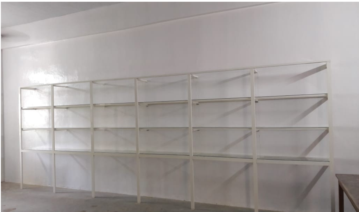
New library in progress
